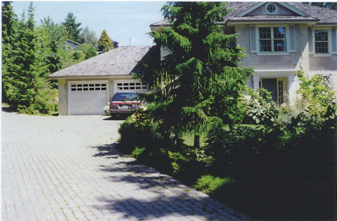
2060 – 2062 Westdean Crescent West Vancouver B.C.
