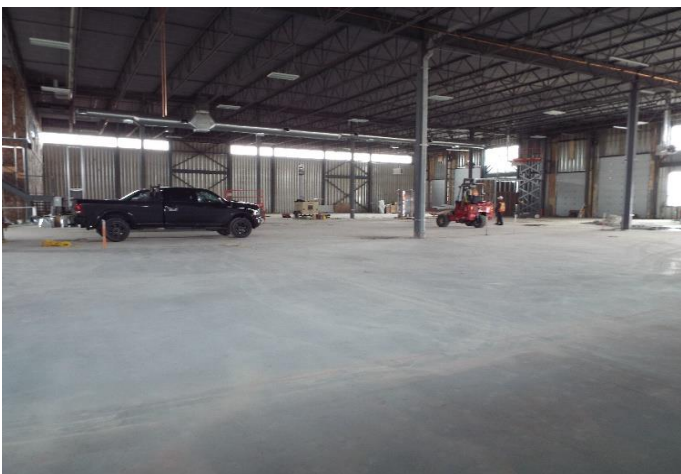
GENERAL VIEW Interior view showing works substantially completed
