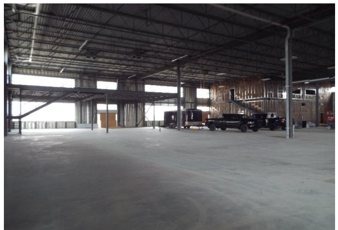
GENERAL VIEW Interior view showing works substantially completed
