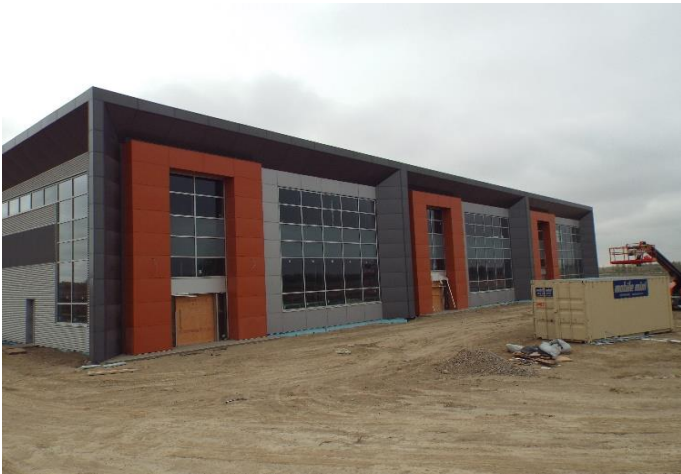
WEST ELEVATION View of exterior enclosure in progress
