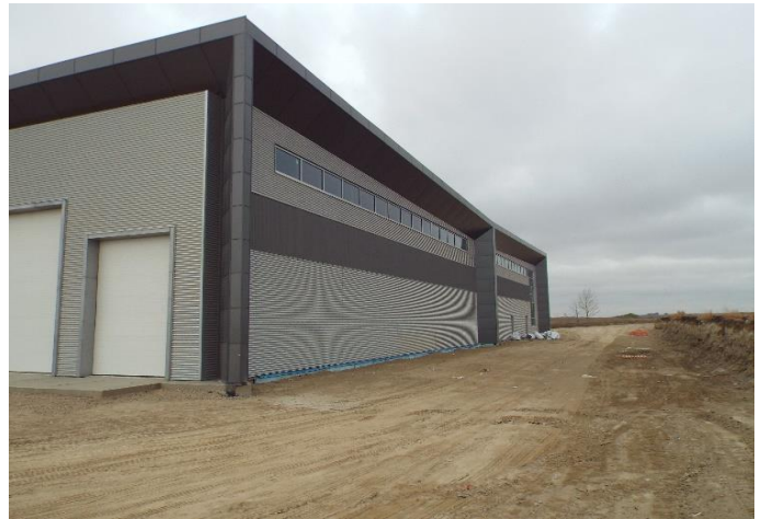
NORTH ELEVATION View of exterior enclosure in progress
