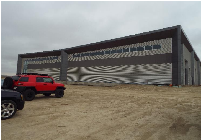
SOUTH ELEVATION View of exterior enclosure completed
