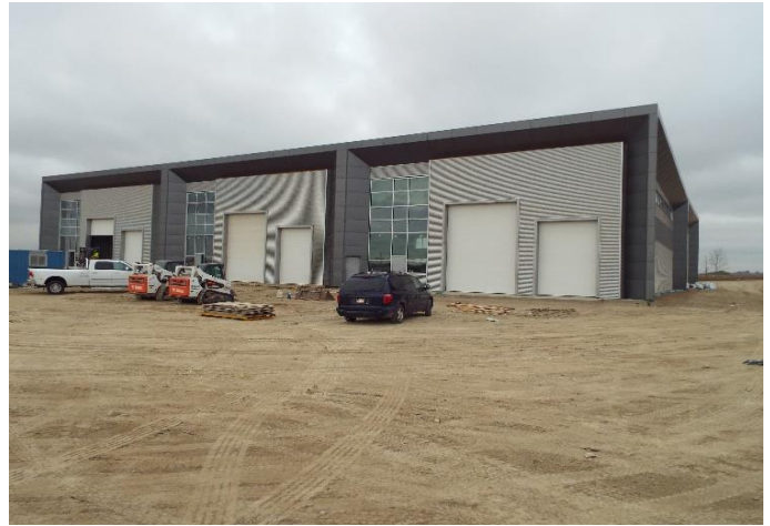
EAST ELEVATION View of exterior enclosure completed
