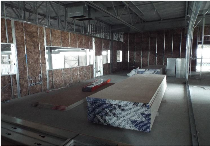
GENERAL VIEW Drywall materials on site
